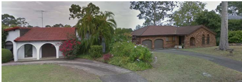
Figure 4 – Single storey houses at 20 & 22 Chapman Avenue, Castle Hill (north boundary of site) Source: Google
