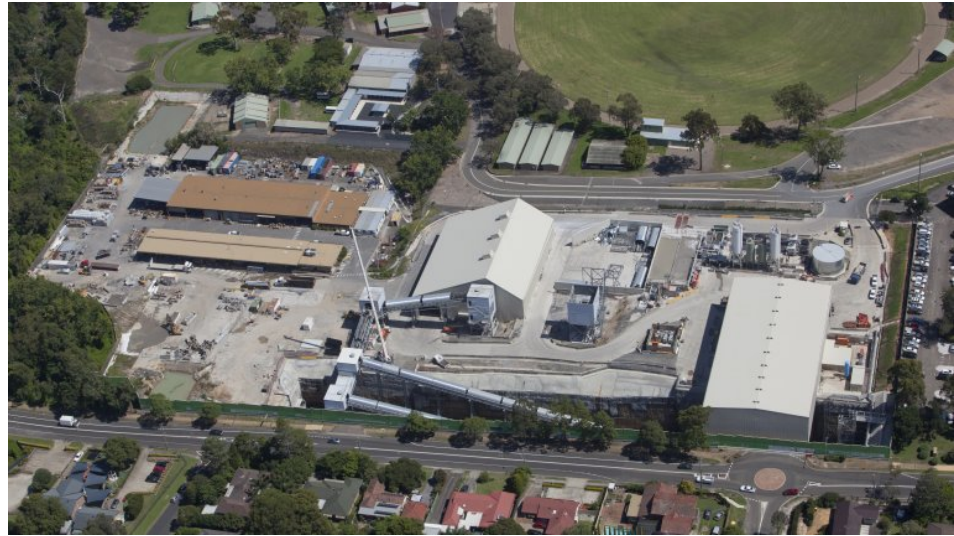
Figure 10 – Aerial view of Showground Station Source: Sydney Metro
